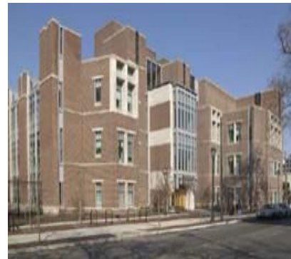
Office building A, USA 6425m 2 , 364kWh/m 2 ·a
