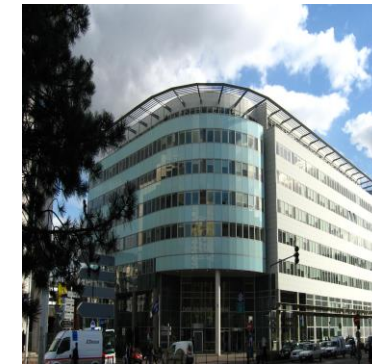
Office building, Lyon 17k m 2 , 165kWh/m 2 ·a
